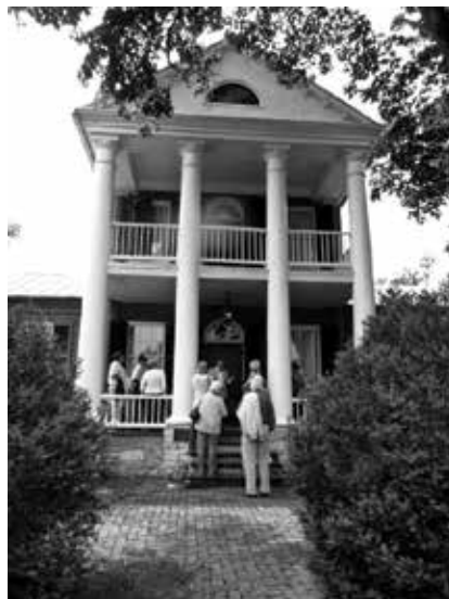
➤ One of Preservation Month's highlights was the tour of Stono, built in the early 1800s by Jordan's Point industrial and transportation entrepreneur John Jordan. VMI Museum Director Keith Gibson led the tour of the property (now known as Turman House), which is rarely open to the public.
