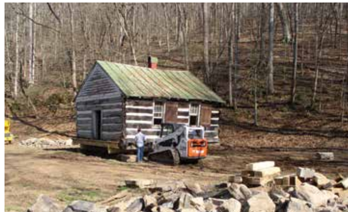
Will and Tommy Harris prepare the Hamilton Schoolhouse for a stone foundation.
