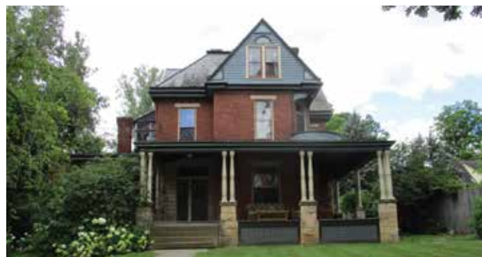
William G. McDowell Home (1891) Queen Anne style shows multi-color wood trim typical of Victorian architecture.
