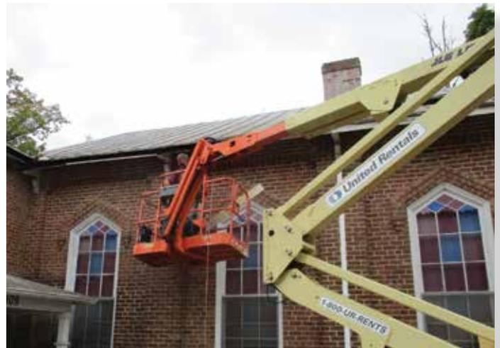
*Welsh Construction workers remove the gutters and replace fascia board in preparation for the installation of new gutters.*
