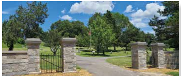
Completed gate and walls at Evergreen Cemetery.
