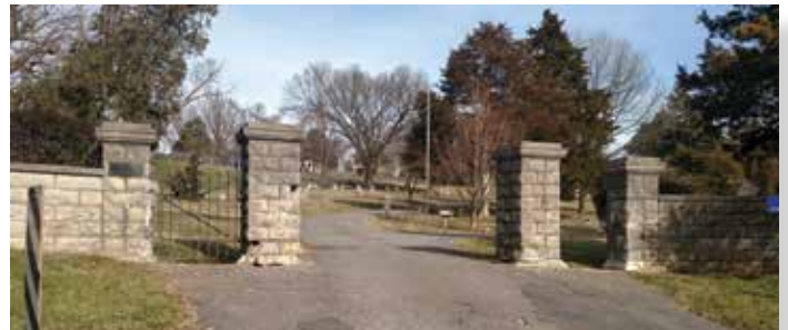
Walls before work commenced at Evergreen Cemetery.
